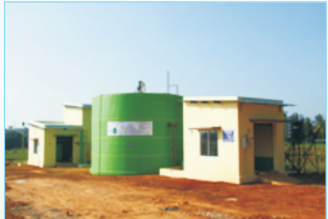
Biogas Generation Unit
